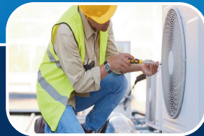
Customized HVAC enhancements
